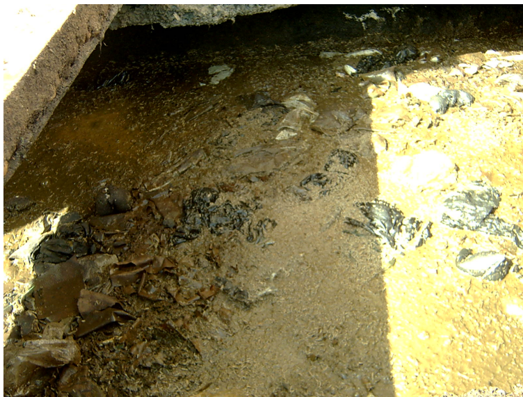
Picture 2: Bulky and inappropriate materials dropped into the pits that can interfere with emptying
